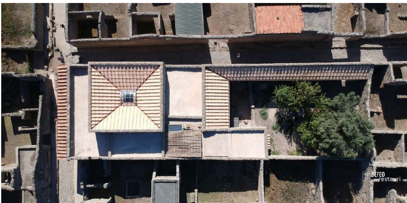
Domus Cerere Pompei post operam copyright de feo restauri
